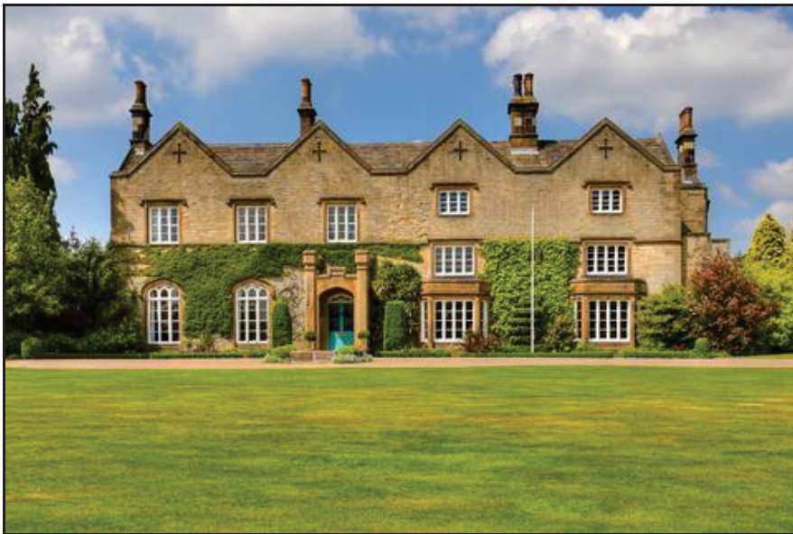
The main front of Dunston Hall. The entrance porch is dated 1826, which is presumably when the present facade was built, but the three-story section to the right appears to be the remains of a typical north Derbyshire 'high house' built by the Milnes family c.1600.
