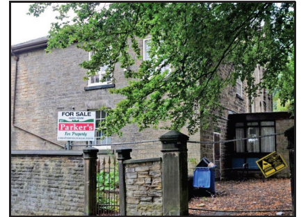
The sadly familiar view of the back of Hurst House, now looking very neglected after being left empty by the county council for seven years. W.T. Parker are no longer acting in the sale of the property.
