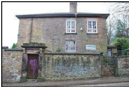
Hurst House: still at risk
